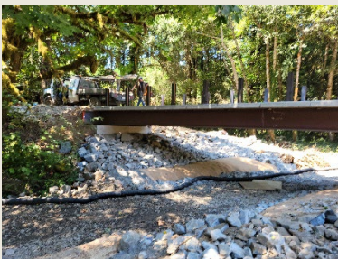
Barrier after bridge
