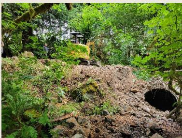
Barrier before bridge
