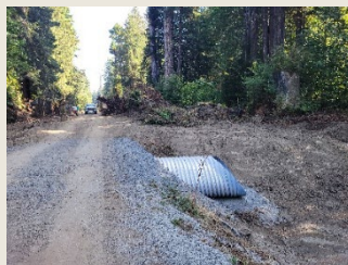
Oxbow inlet culvert
