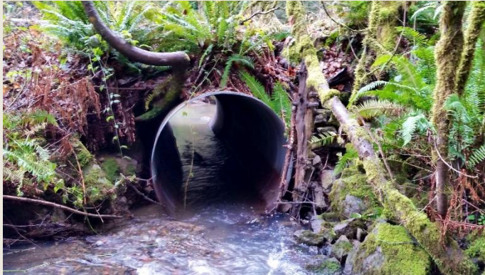
View looking downstream at culvert inlet.
