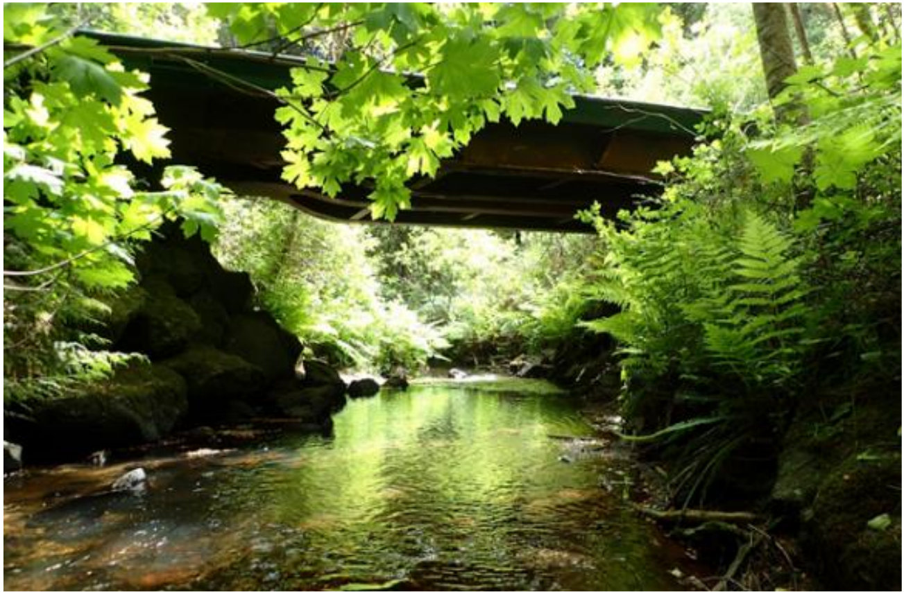
Bridge over Lindsay Creek
